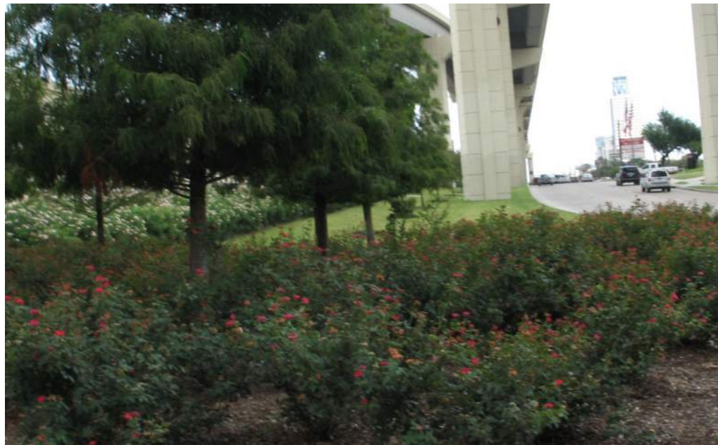
Beltway 8 and I-10 Interchange
